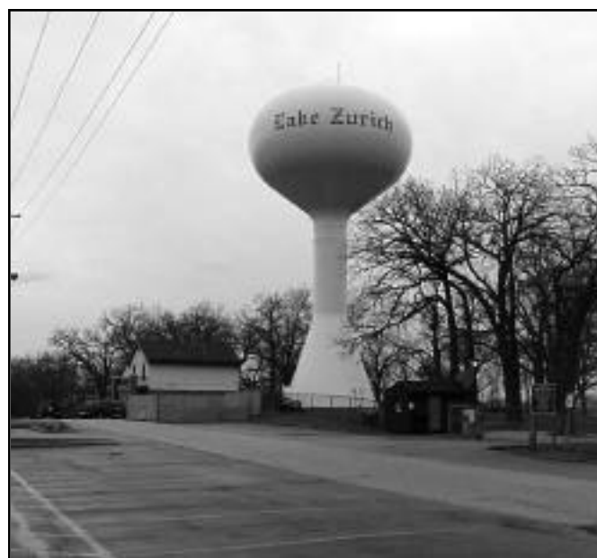
The 750,000 gallon elevated storage tank at Paulus Park.
